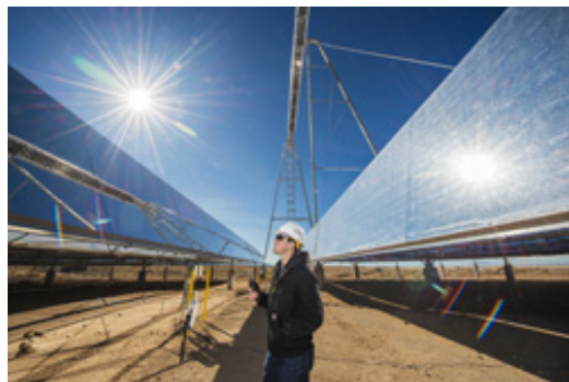
Steve Sellers of AREVA Solar stands amid the Compact Linear Fresnel Reflectors, the mirrors that focus sunlight to the top of the structure where molten salt is flowing. The resulting heat is stored and used later when the sun is not shining. (Photo by Randy Montoya) Click on the thumbnail for a high-resolution image.
