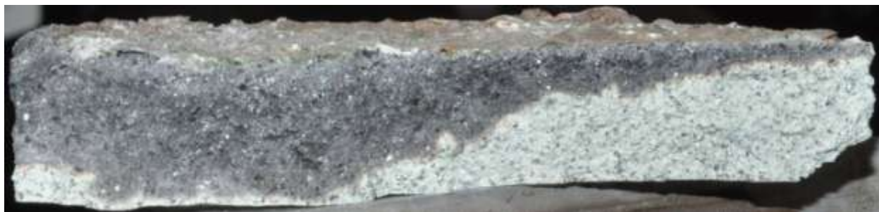
Figure 54. Cross section of the clay bonded SiC base plate used in the high temperature furnace. Affected areas are discolored black with some associated swelling.
